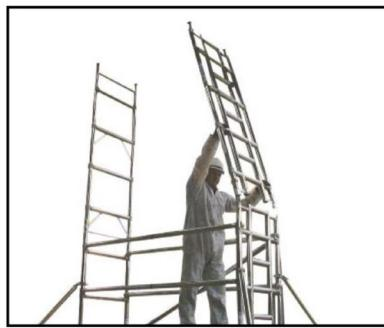
8. To add further frames, stand on the platform disengage your interlock clips and add your frames on top of the spigots ensuring the ladder is continuous.
