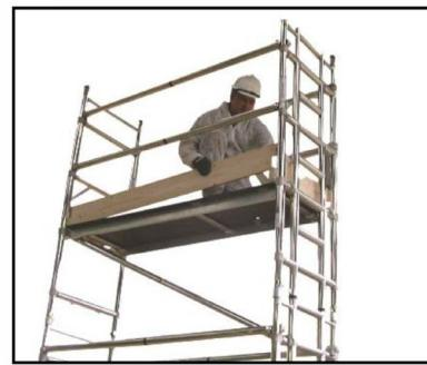
13. Fit toe-boards in the correct position.
