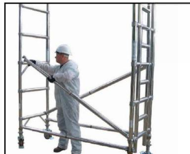
4. Facing the plain frame fit 1 diagonal to the bottom rung as close to the right hand frame vertical as possible. Facing the ladder frame fit 1 diagonal to the bottom rung as close to the ladder as possible.
