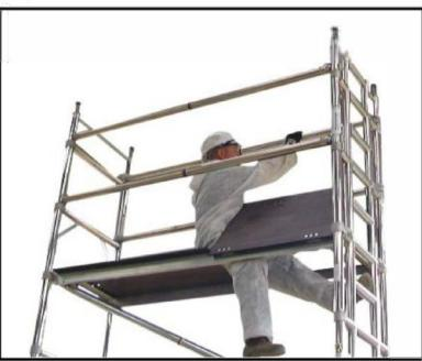
12. From a seated position, using the through the trapdoor (3T) method, fit four horizontal braces above the appropriate rungs to the frame verticles. Hooks facing out.
