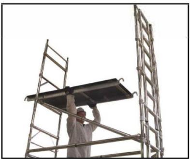
11. Facing the plain frame, fit a trapdoor platform on appropriate rung\* over the brace hook as near to the frame verticle as possible, trapdoor to ladder frame end (\*see base set up Fig 1 guide).
