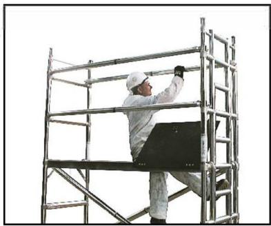
6. From a seated position, using the through the trapdoor (3T) method, fit four horizontal braces above the appropriate rungs to the frame verticles. Hooks facing out.
