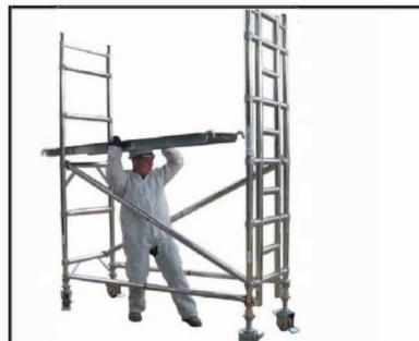
5. Facing the ladder frame, fit a trapdoor platform on appropriate rung\* inside the brace hook as near to the ladder as possible.
