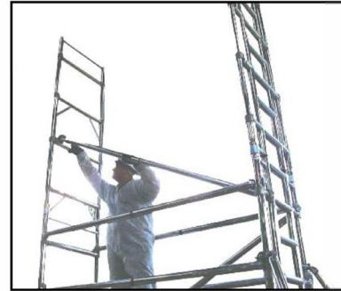
10. Fit diagonal braces to continue in a regular pattern from rung to rung except when interrupted by an intermediate trapdoor platform.
