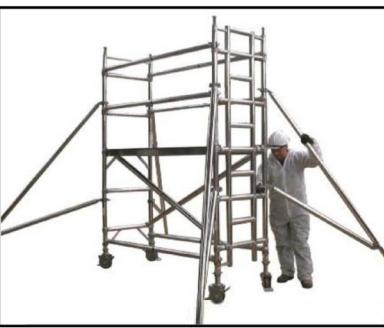
7. Secure stabilisers as soon as possible to increase tower stability. Check tower kit list to ensure the correct stabilisers are fitted.
