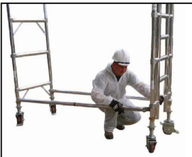
2. Fit in 2 horizontal braces to the vertical member of the frames, as low as possible, below the 1st rung. All horizontal braces fit on from inside the tower facing out.
